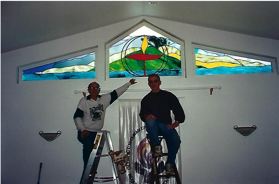
2005 installing window Forest Davis & Jerry Fryrear
